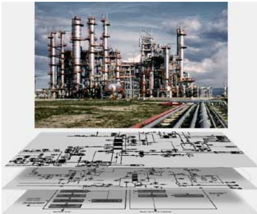
A view of a refinery plant [6].
